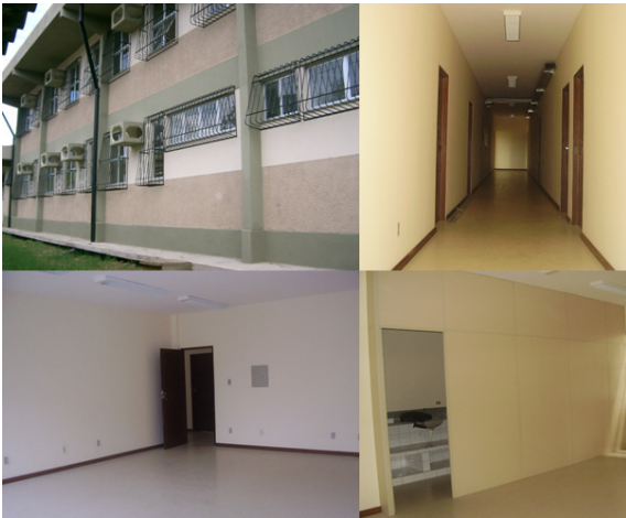
Fig. 1. From up left clockwise: front of building, second floor corridor; room separated by wall, and room separated by brick wall.
